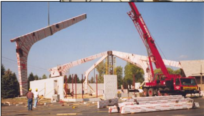
(Crane:) A crane swings one of the enormous church beams into position. The crane was rented for 14 hours!
